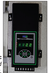
Photo A: When installing or servicing, hang by two screws, to support the controller. shown wired using the Wire Harness.
